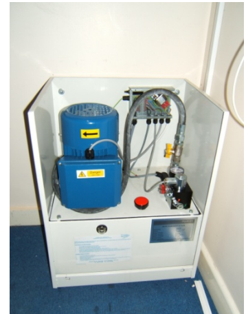
Hydrax pump unit which uses a square key. Stannah part no.555800
